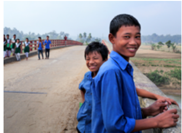
Children going to school using Mahalchari bridge over the Chengi River. The bridge was built in 2009 under the Chittagong Hill Tracts Rural Development Project by ADB. Photographer: M R Hasan
