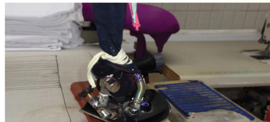
After-Installation of Steam Traps
