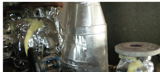
After-Insulation of bare hot surfaces
