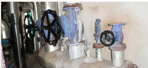
Before-Insulation of bare hot surfaces
