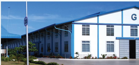
Buildings are designed to provide natural ventilation through louvers near ground level and vents along the roofline and the ridgeline.
